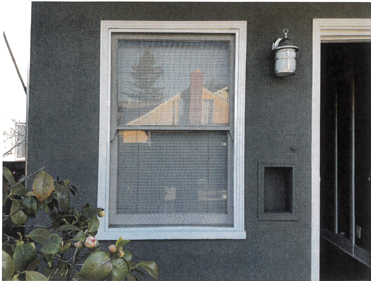
Window 7 – Back porch window. Kitchen on interior.
