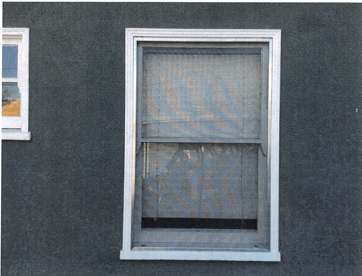
Window 2 – Bedroom window
