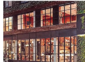
4 STEEL SASH STOREFRONT WINDOWS
