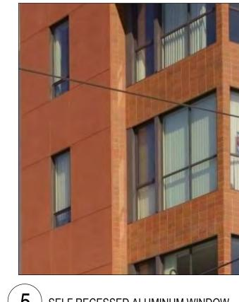
5 SELF RECESSED ALUMINUM WINDOW SYSTEM - CLEAR ANODIZED WITH CLEAR AND OPAQUE GLAZING
