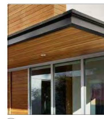
11 METAL ENTRY CANOPIES, WITH WOOD SOFFIT
