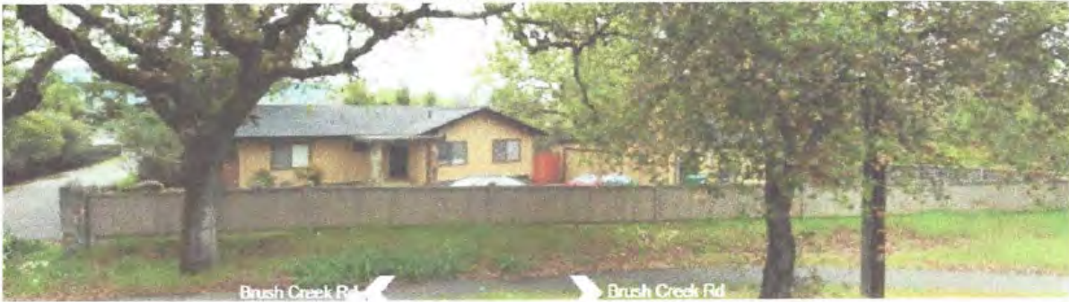
Before Photo showing Dirt Between Fence and Sidewalk on Scenic Brush Creek Road
