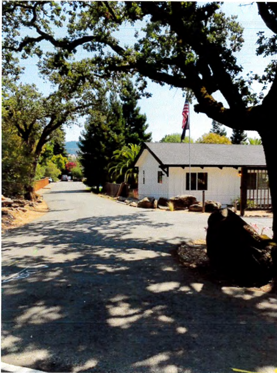
View into driveway as of July 31, 2020 from scenic Brush Creek Rd.
