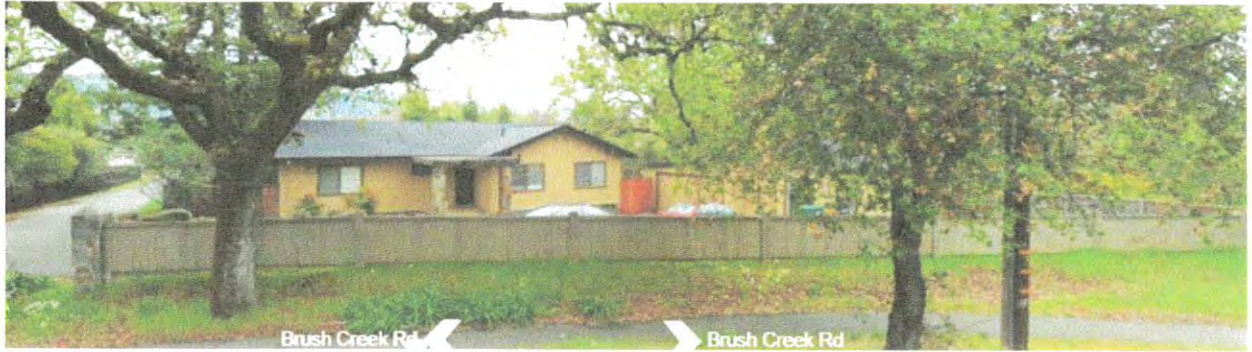
Before Photo showing Dirt Between Fence and Sidewalk on Scenic Brush Creek Road
