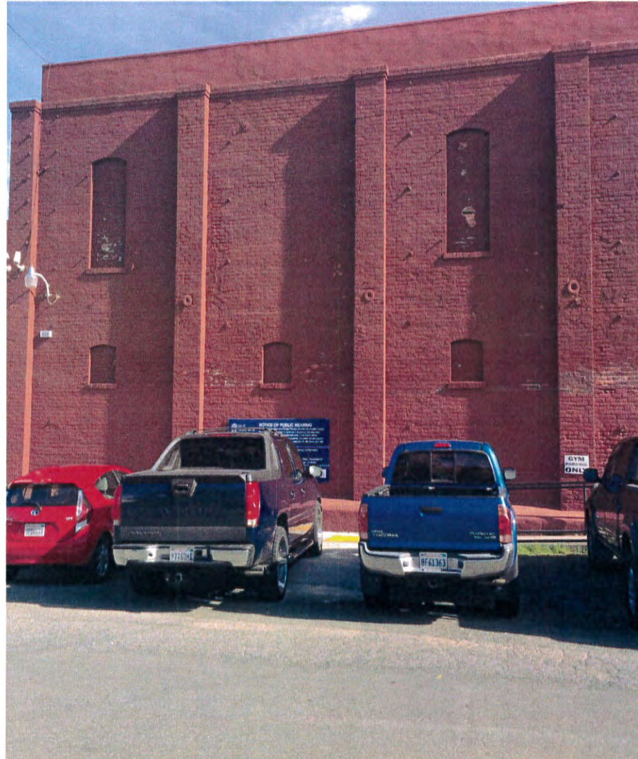
Up-close view of Donahue Primary wall.
