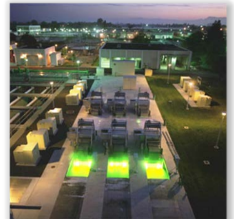
Laguna Treatment Plant
