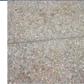
PAVEMENT ONE CONCRETE SCORING: SAWCUT FINISH: EXPOSED AGGREGATE COLOR: INTEGRAL COLOR, TBD.
