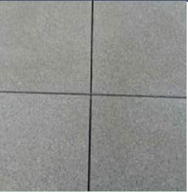
PAVEMENT ONE CONCRETE SCORING: SAWCUT FINISH: GRACE TOP CAST SANDBLAST COLOR: FEWTER, DAVIS COLORS
