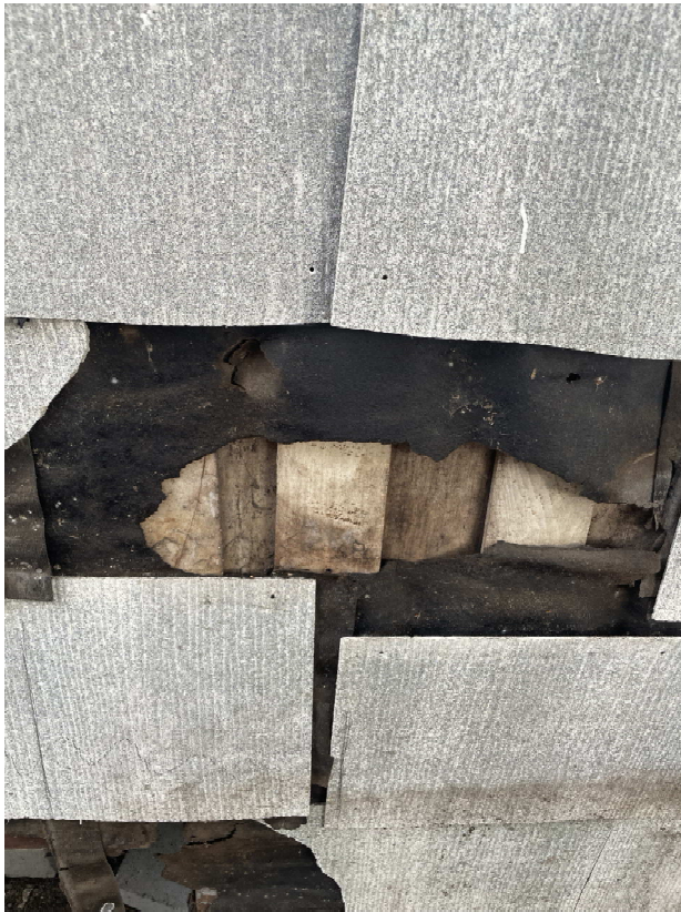
Exposed original siding details
