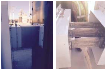
Figure 8: An illustration flex cable connecting the transformer to the inverter
