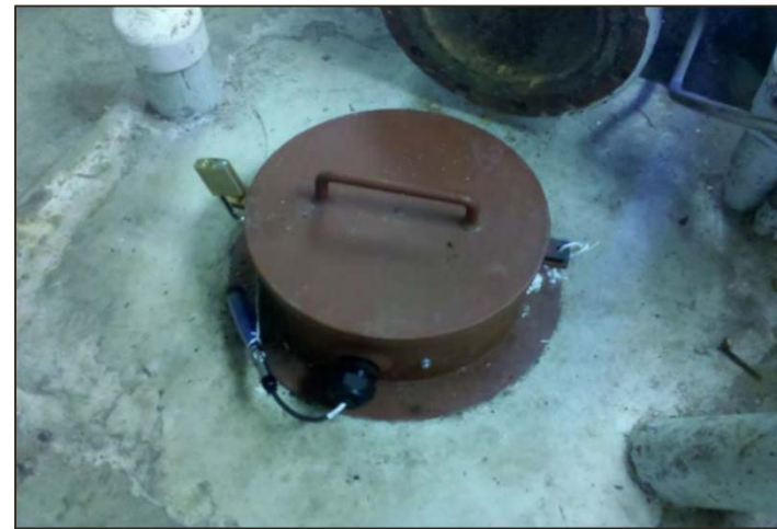
Freeway well surface enclosure with transducer and desiccant pack
