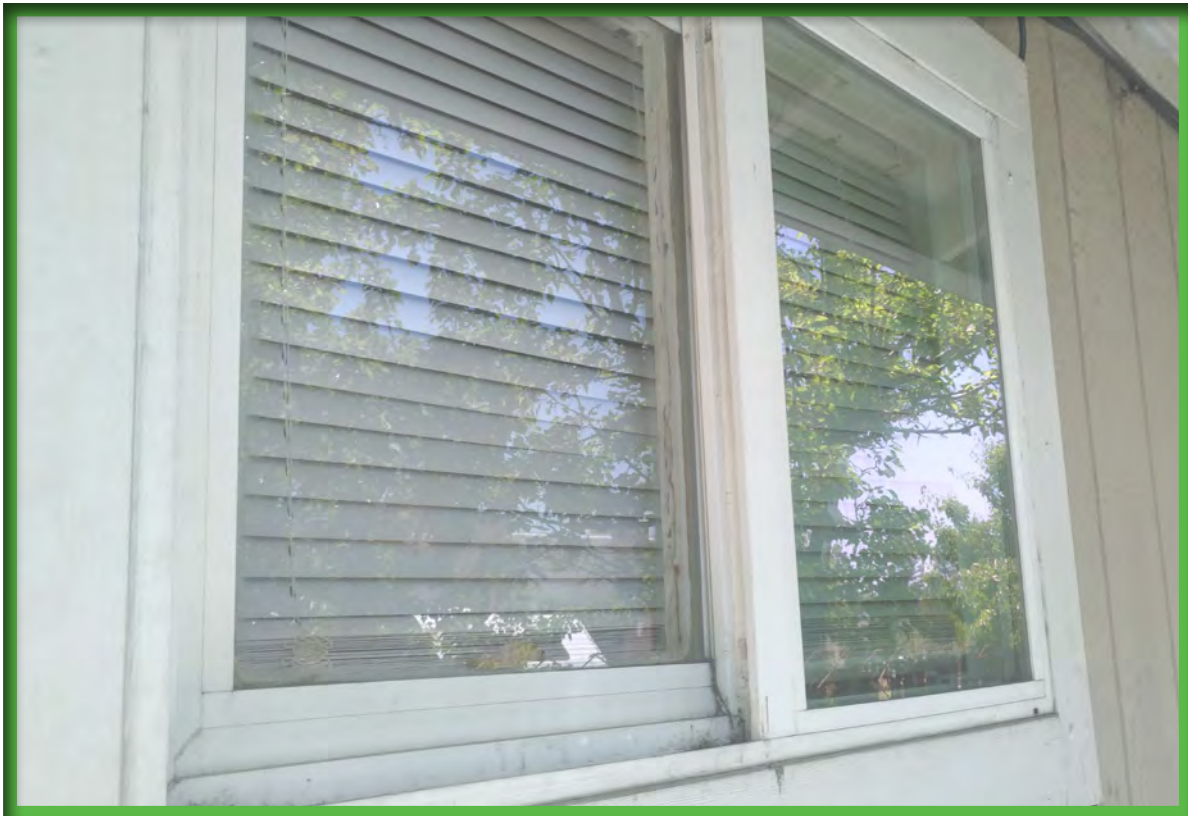
H. Newly Installed Dual Pane Windows in Good Condition with Minimal Maintenance Issues (Permit for Inserts Not Required)
