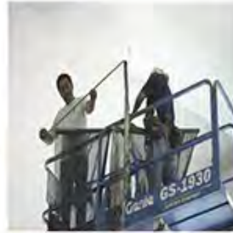
Measure, square & tighten tubes
