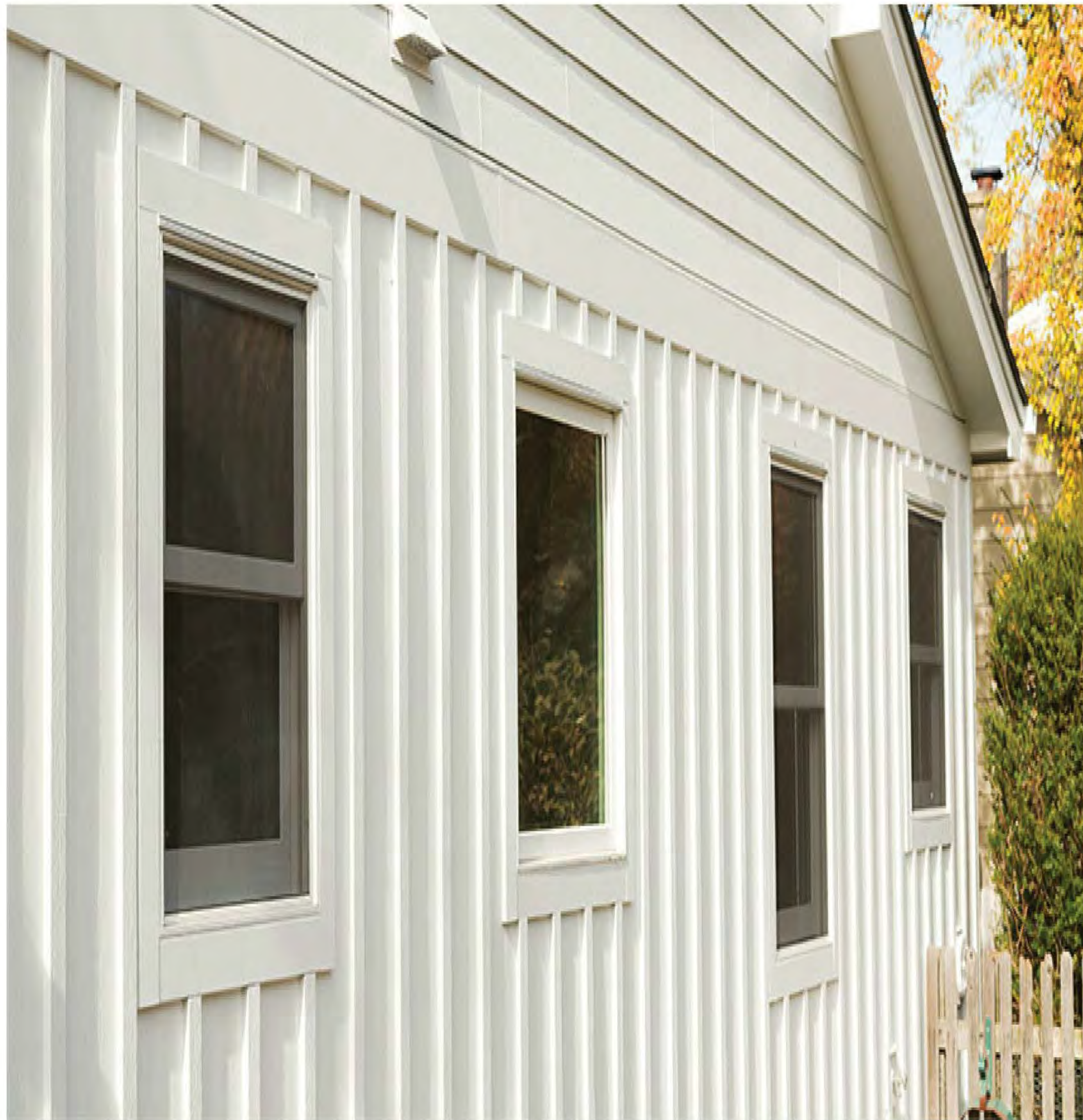
HARDIEPANEL VERTICAL SIDING BOARD AND BATTEN
