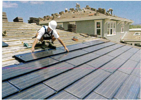
Figure 4.10.31 Integrated solar panels.
