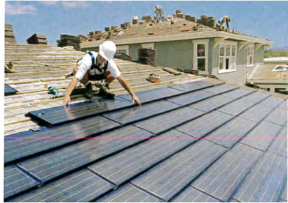
Figure 4.10.31 Integrated solar panels.
