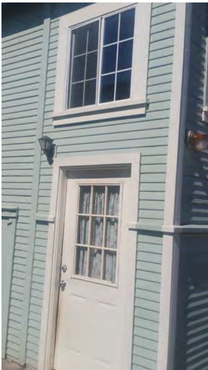
False divided light and door to be removed.
