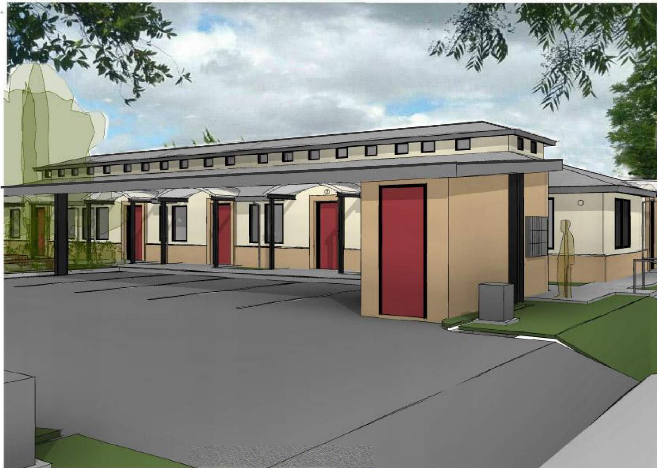
South Building North View
