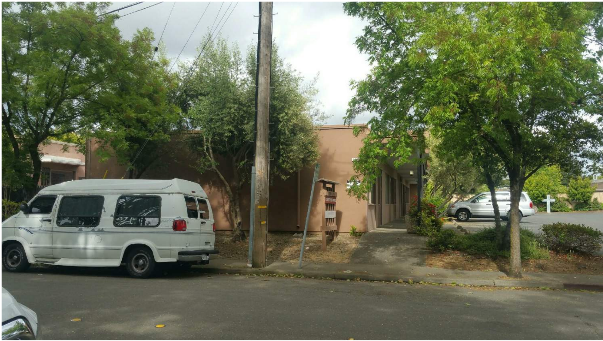
North Building McBride Lane View
