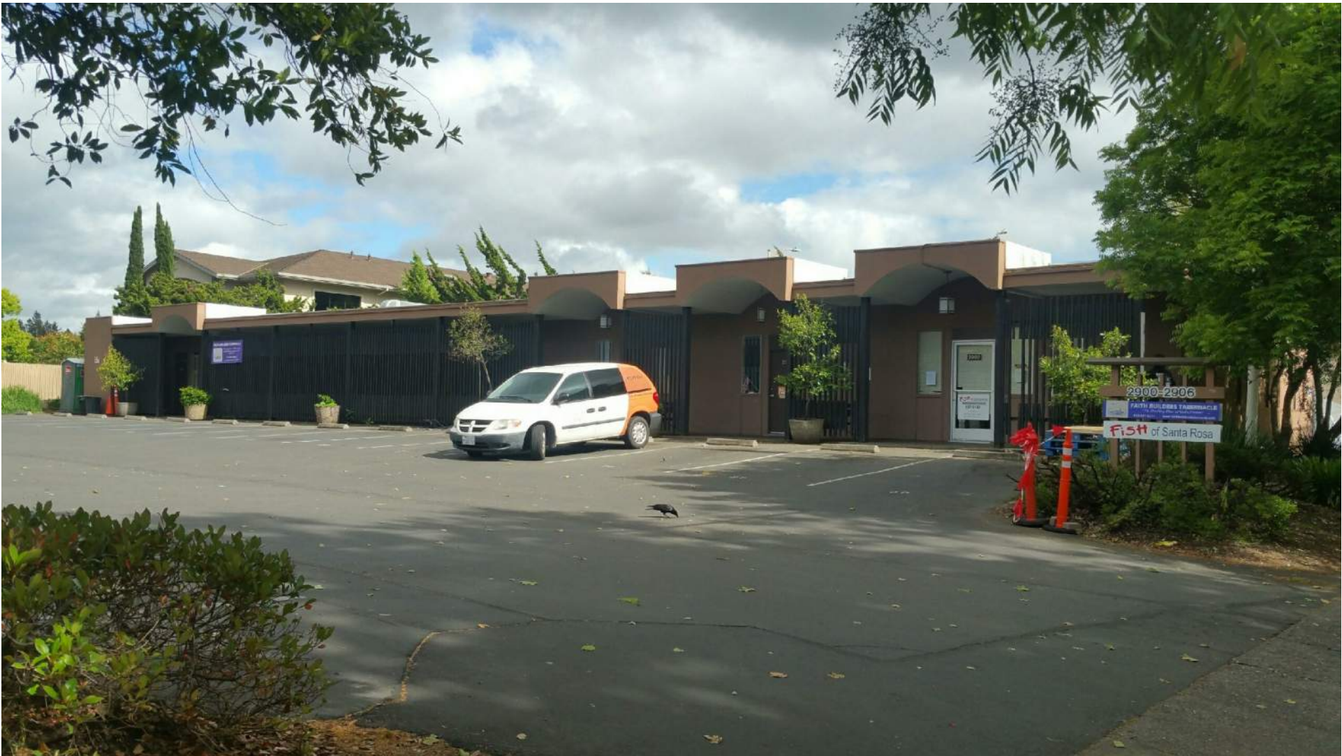
South Building North View
