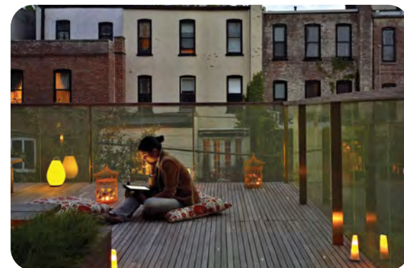
Wood Decking and Glass Guardrail
