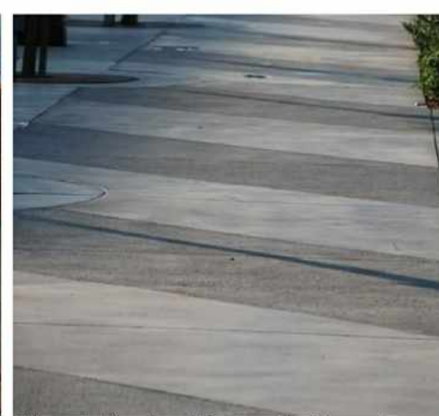
Alternate Bands of Permeable Concrete and Impervious Concrete
