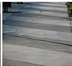
Alternate Bands of Permeable Concrete and Impervious Concrete
