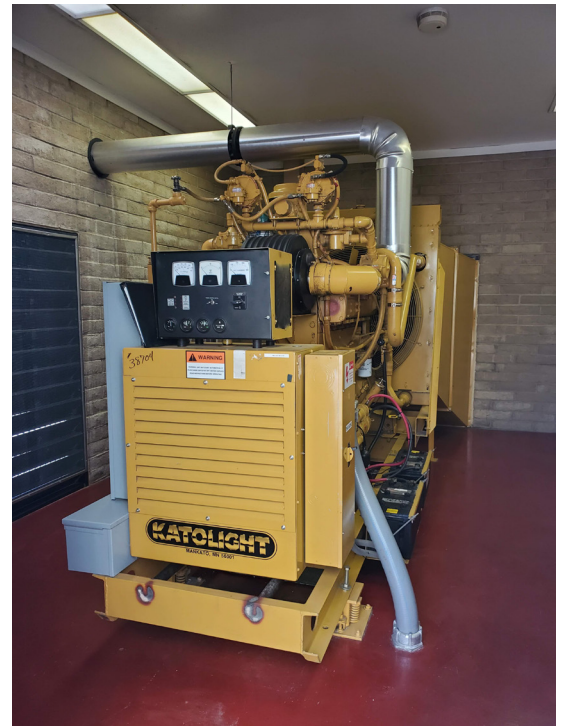
Existing 150kw generator set at S-17. Replacement generator will be significantly larger capacity and may not fit into existing space.
