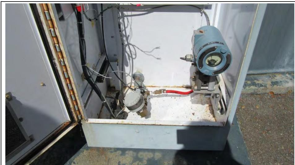
**Photo 25. Reservoir R-3 Pressure Transmitter**
