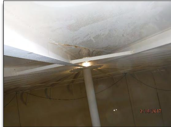
Photo No. 8 – Interior roof view of R-17 with minor corrosion on roof seams.
