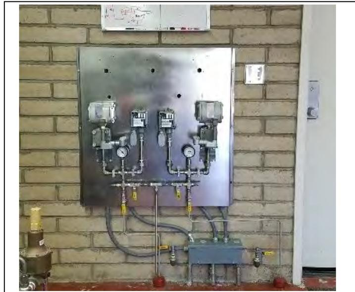
**Photo 11. Pump Instrument Panel**
