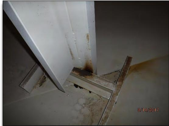
Photo No. 14 – Interior of R-9A with minor corrosion at seams.
