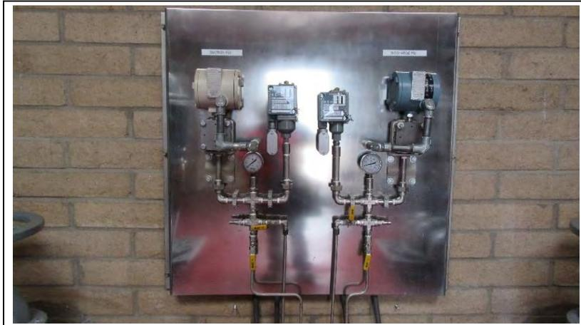
**Photo 22. Pump Instrument Panel**
