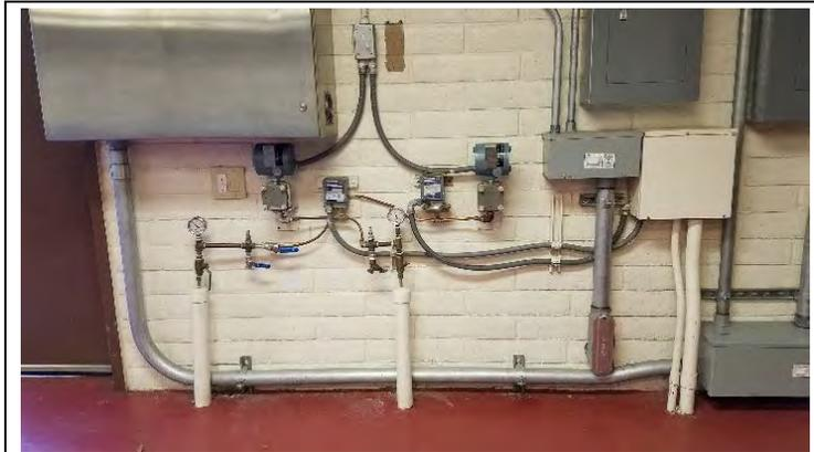
**Photo 6. Pump Instrument Panel**
