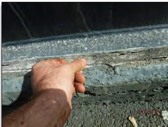
Photo No. 17 – R-9A annular ring with sealant between annular space and concrete pad.
