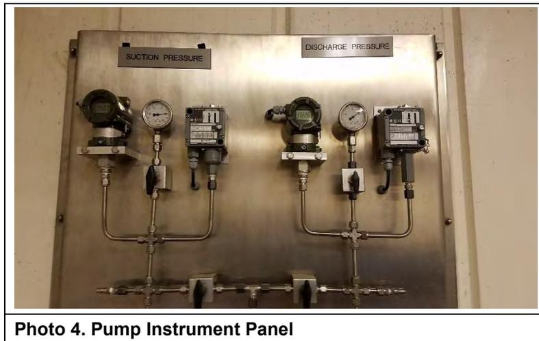
Photo 4. Pump Instrument Panel
