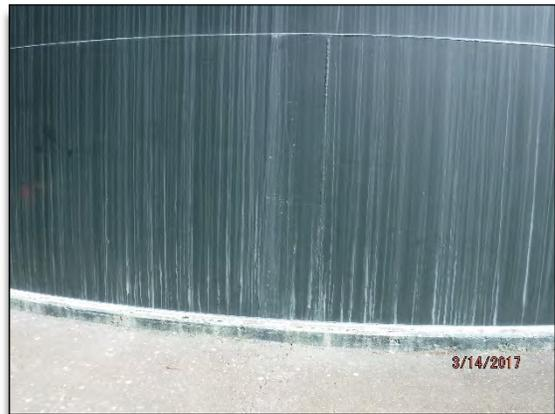
Photo No. 16 – Exterior of R-9A with chalking present on exterior coating.
