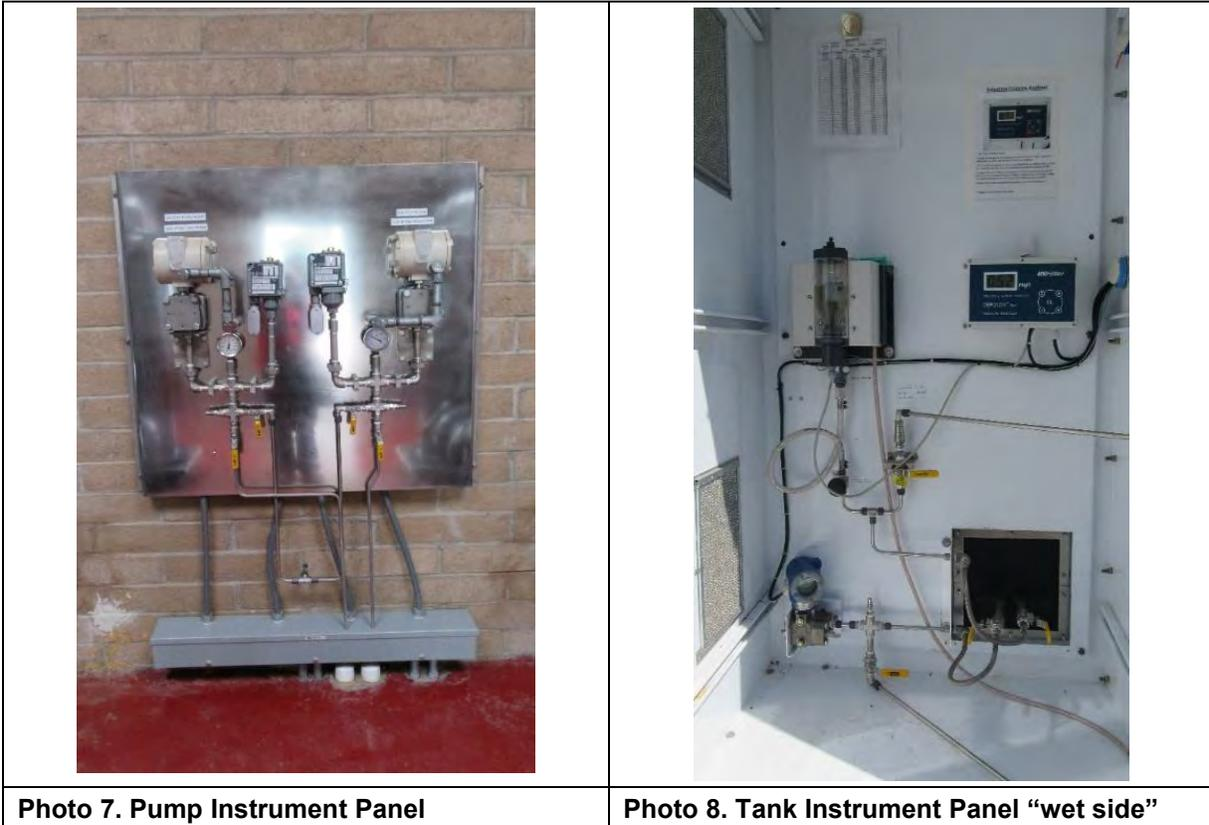
The R16 tank is monitored by a L2000 PLC with small form factor LED Operator Interface. The PLC is provided with battery backup with battery charger in the event of power failure.
