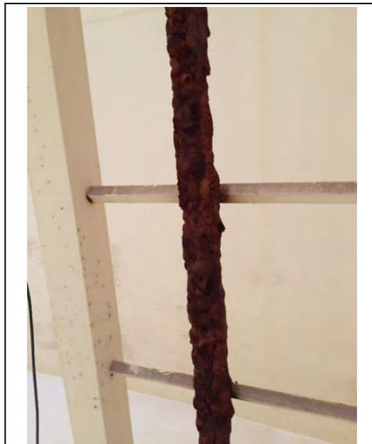
**Photo 2-4. Interior Ladder Saf-T-Climb with Corrosion Product on the Surface**
