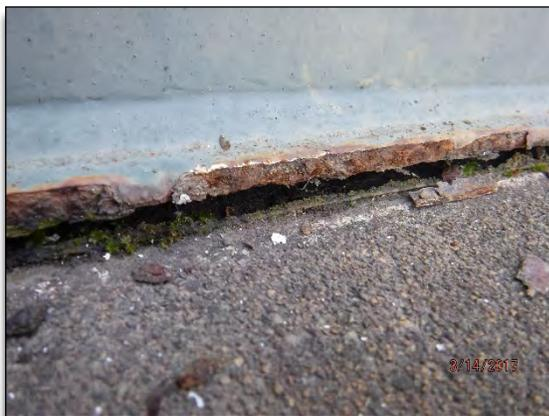
Photo No. 5 – Annular ring wall with moss growing under tank.
