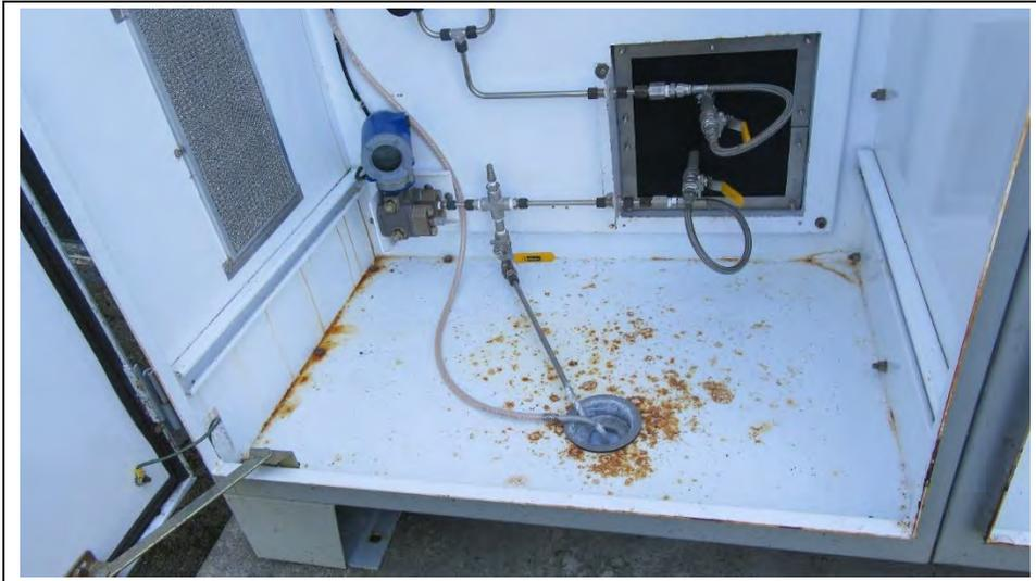
**Photo 1. Reservoir R-9A Tank Sampling Equipment**
