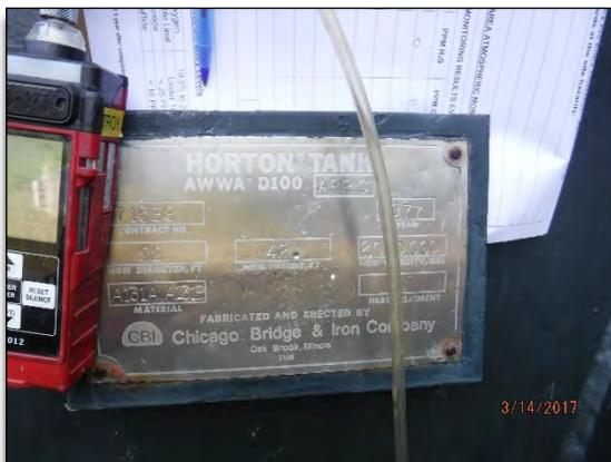
Photo No. 11 – Horton Tank R-9A identification plate.
