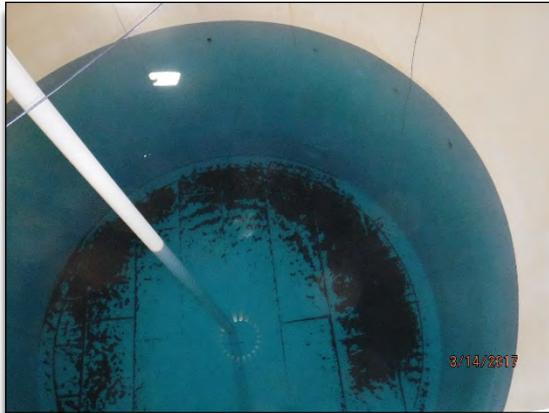
Photo No. 7 – R-17 interior view with debris on bottom.
