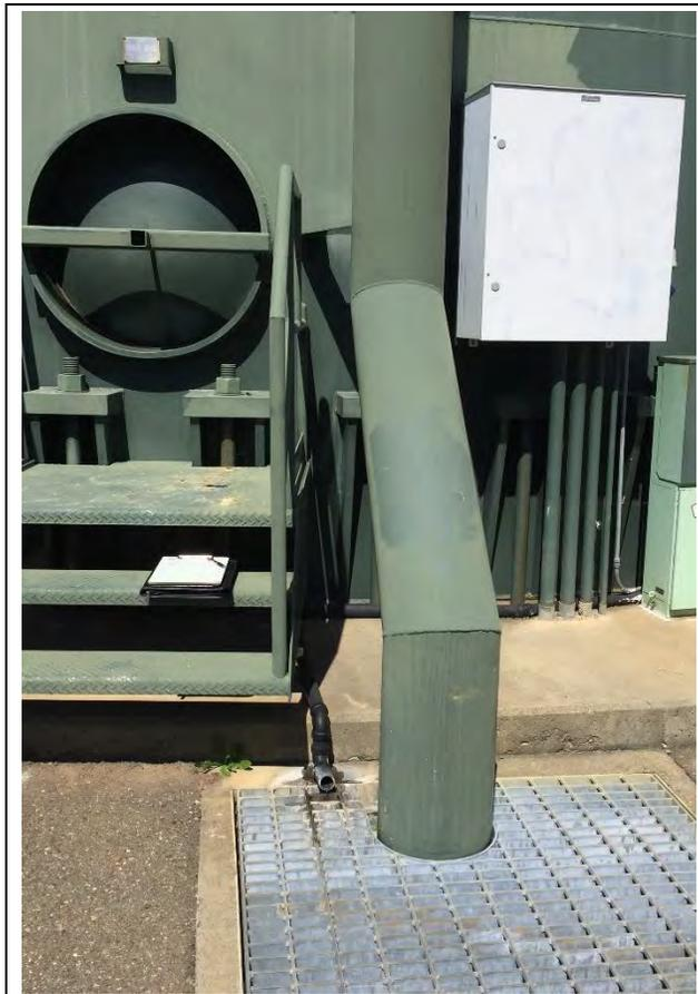
**Photo 4-2. Reservoir R-17 Overflow Direct Connection to the Storm Drain System**
