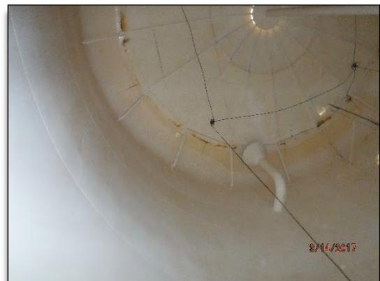
Photo No. 4 – Interior view of R-16 with anodes still suspended from ceiling.
