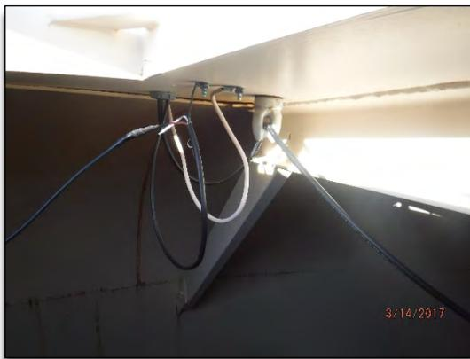
Photo No. 3 – Remains of abandoned cathodic protection system on R-16.
