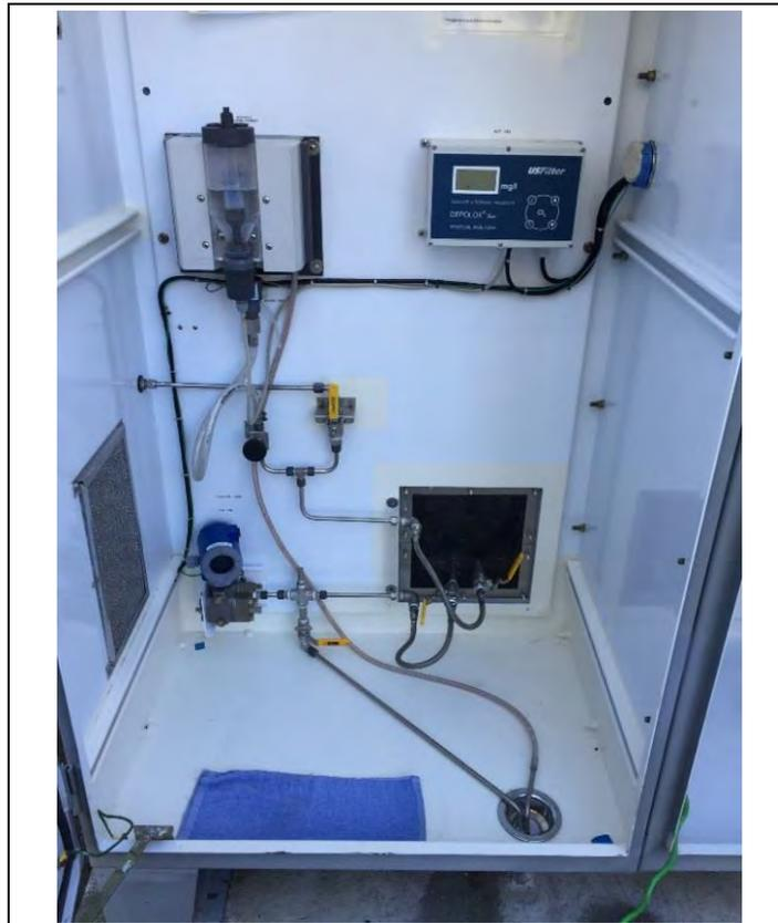
Photo 3-1. Reservoir R-16 Tank Sampling Equipment
