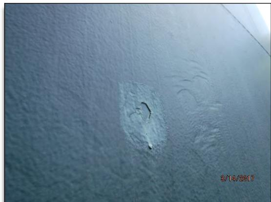
Photo No. 18 – Exterior coating repair of R-9A likely from rock damage.
