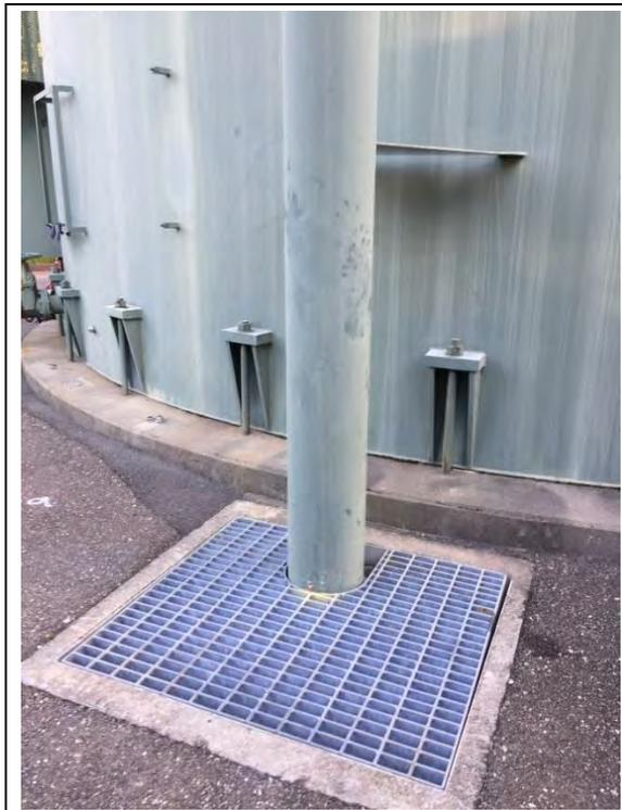
**Photo 3-2. Reservoir R-16 Overflow Direct Connection to the Storm Drain System**
