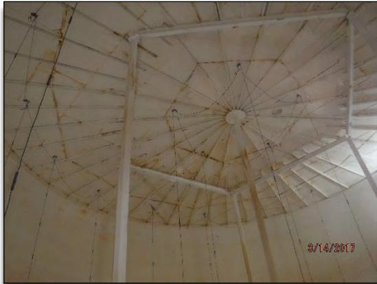
Photo No. 13 – Interior of R-9A with anodes still suspended from roof.
