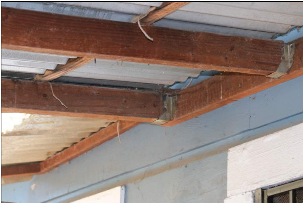
Junction of roof covering with house
