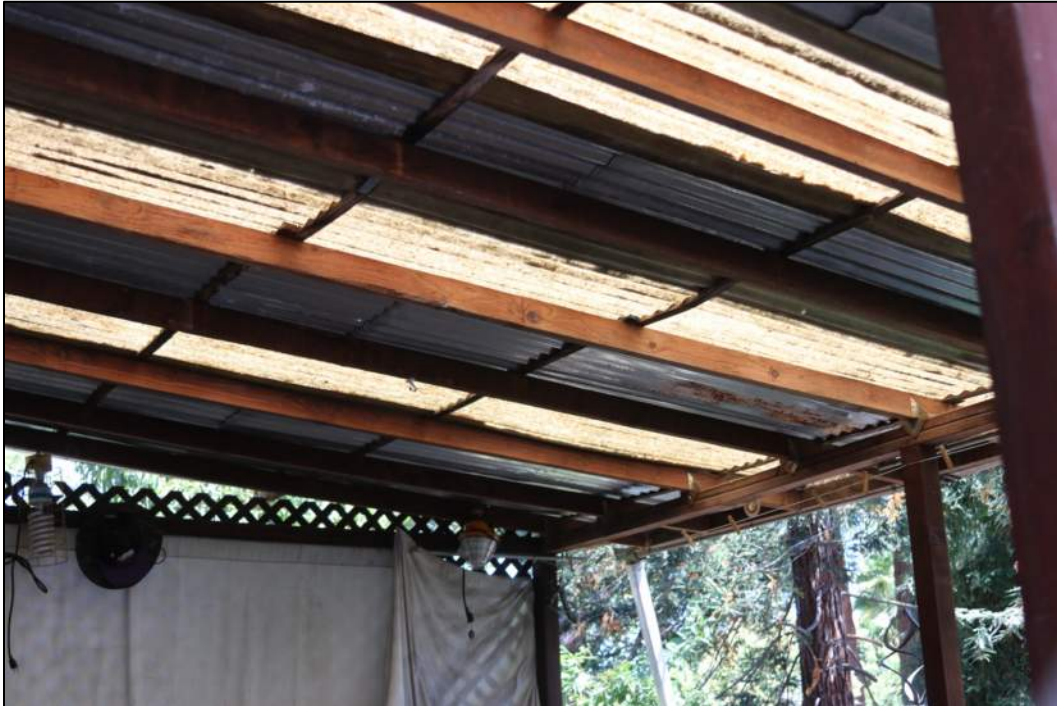
Corrugated metal and plastic covering over deck
