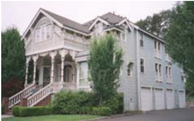
A reconstructed building in the St. Rose Preservation District retains the original façade elements while new construction to the rear provides units in the downtown area.
