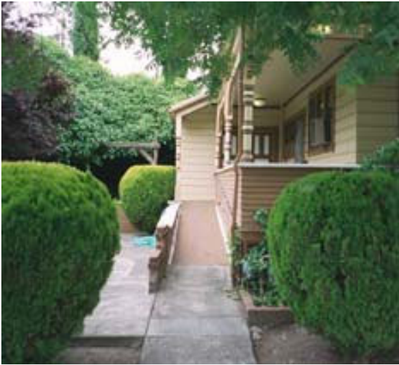
Access ramp is located to the rear of this Queen Anne house (listed in the National Register) which is now used as an office.
