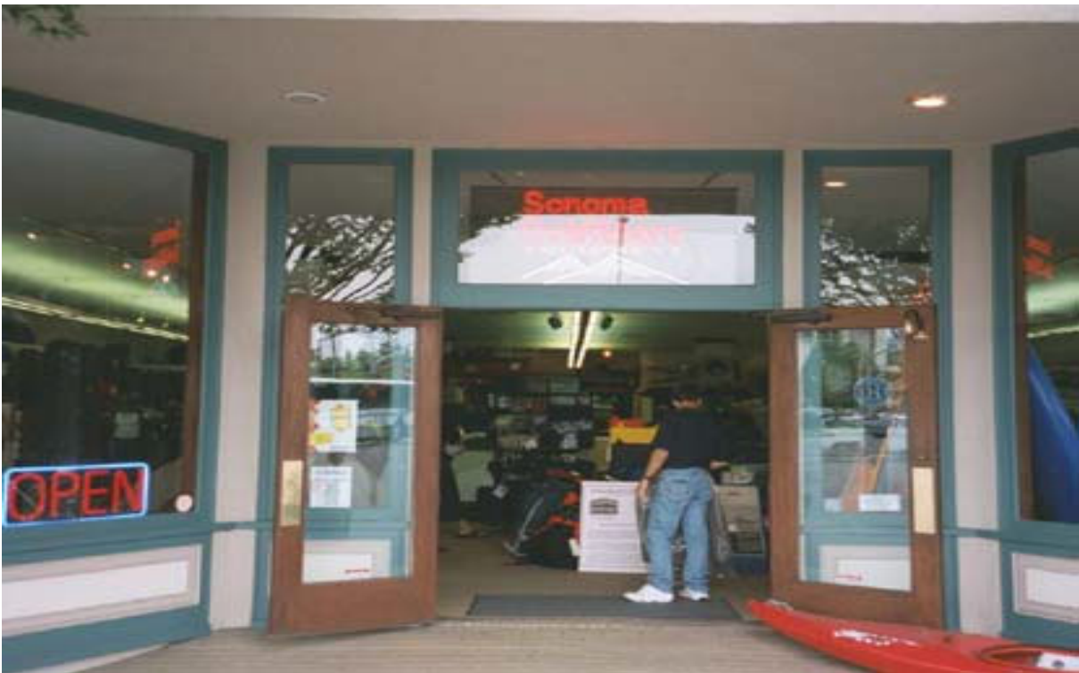
New storefront in the Railroad Square Preservation District “reads” as a traditional storefront.
