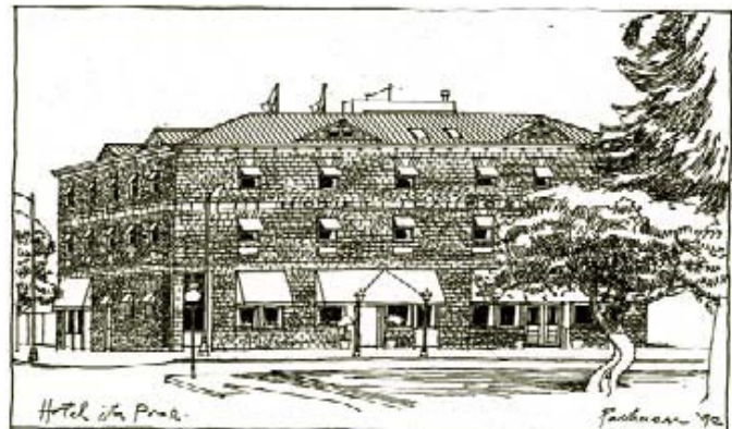
Three-story basalt stone building. – Railroad Square
