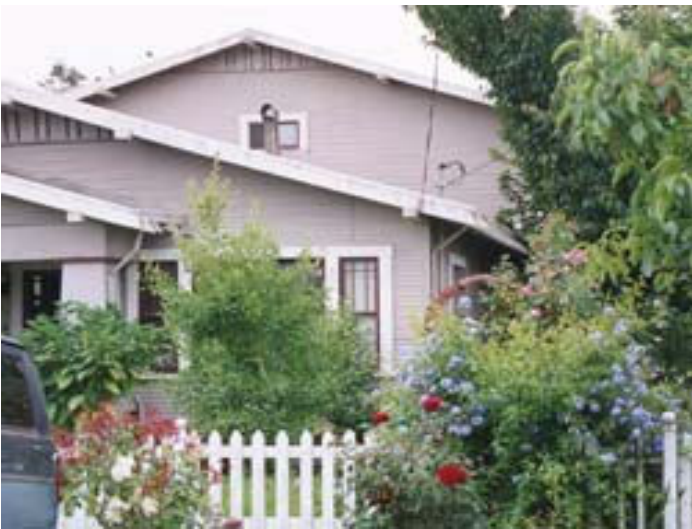
A second-story addition to this St. Rose Bungalow has been set back from the existing building front.
