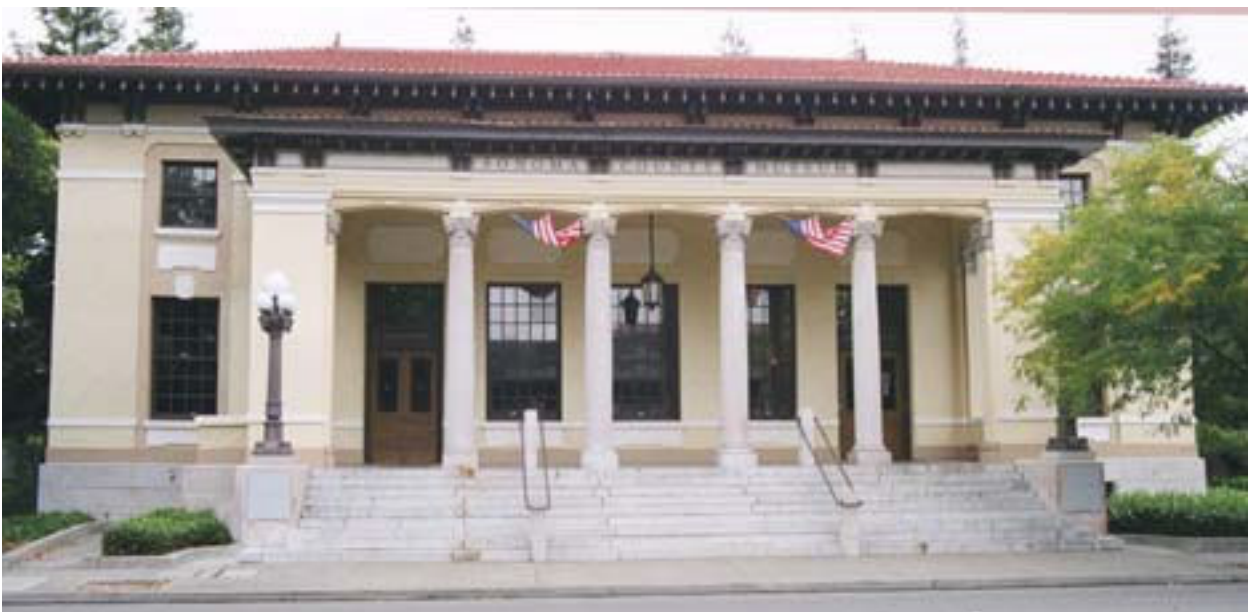
The old Santa Rosa Post Office, a Roman Renaissance Style building, was moved from its Fifth Street site (in a Redevelopment area) to its current Seventh Street location in the St. Rose Preservation District. The restored landmark houses the Sonoma County Museum.
