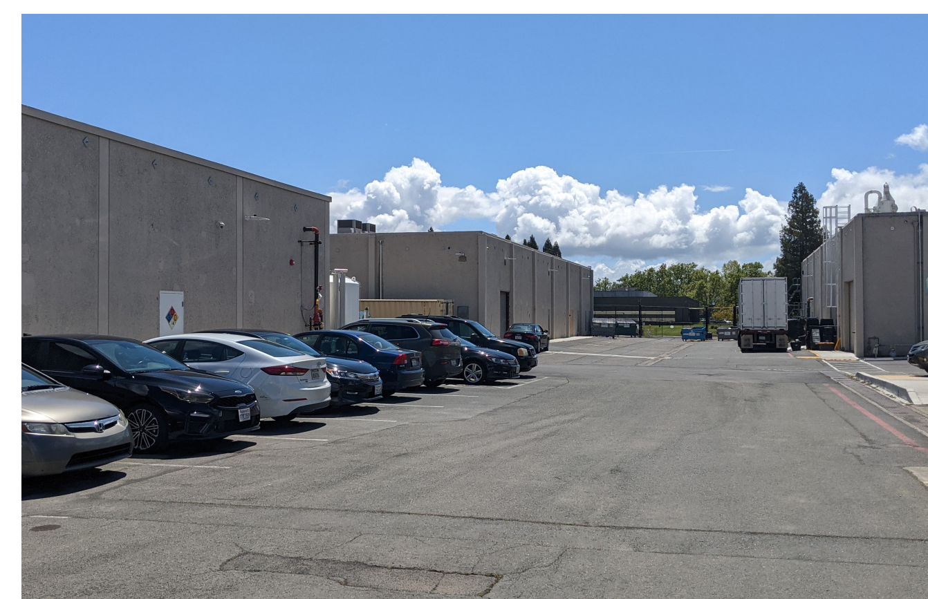
IMAGE 10 / EXISTING BUILDINGS 4, 5, AND 7
