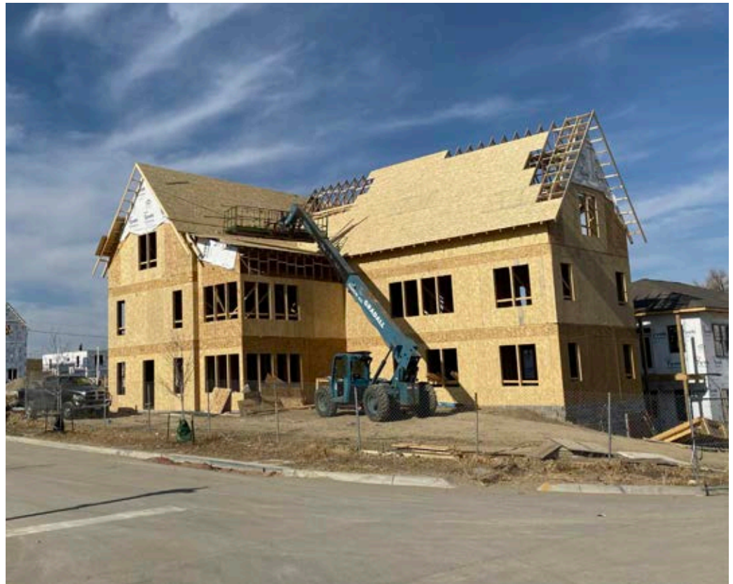
Figure 2.6 The simple forms, smaller size, and compatibility with Type V construction help maximize affordability and investment returns, and are consistent with the construction strategies familiar to most residential homebuilders, as shown in this under-construction MMH project in Papillion, Nebraska.
