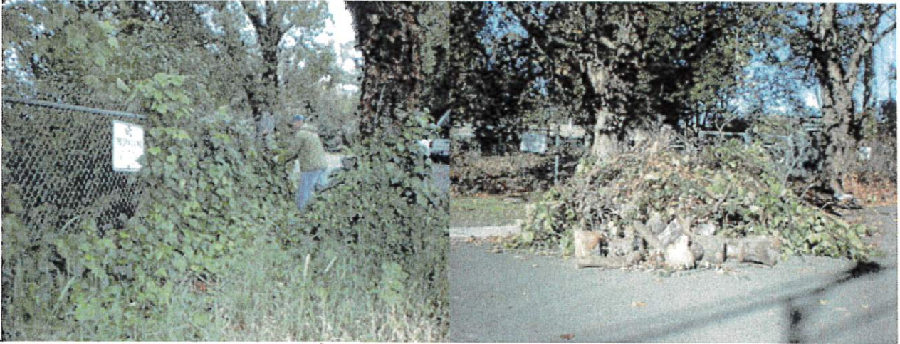
Cal Tran removed the chainlink
