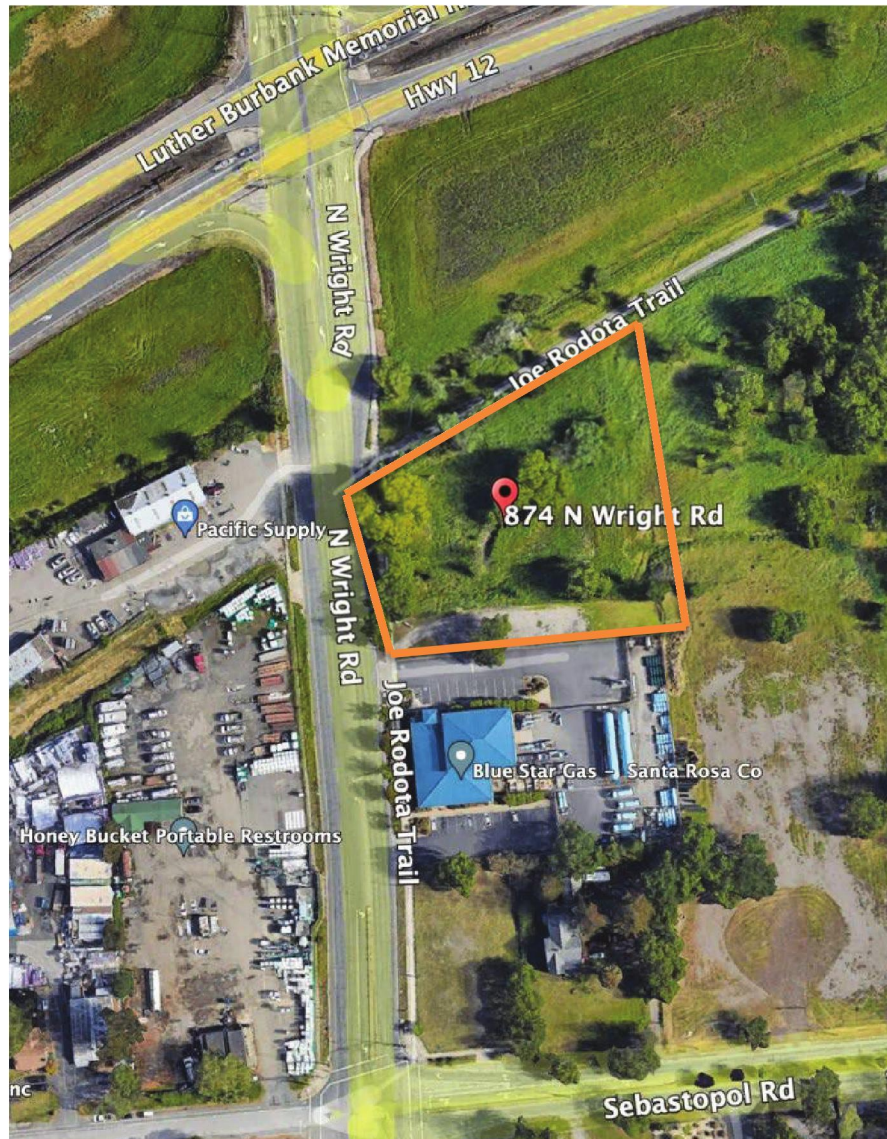
Figure 2: Project Site – Existing Conditions
