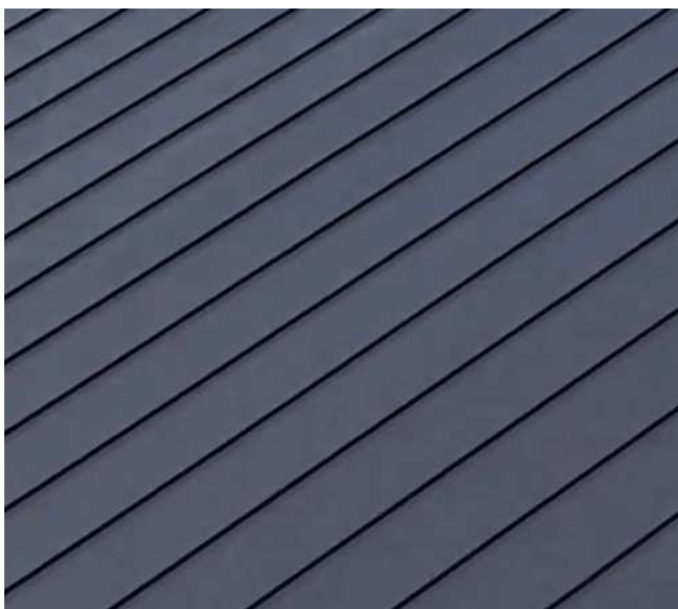
J. STANDING SEAM - SUNSHADES & CLUBHOUSE ROOF
