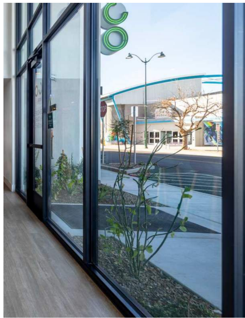
E. CLEAR GLAZING IN DARK ALUMINUM STOREFRONT
