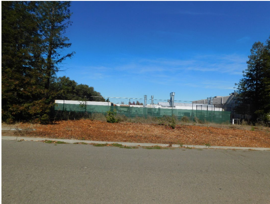
1. Photo facing north towards the parent property.
