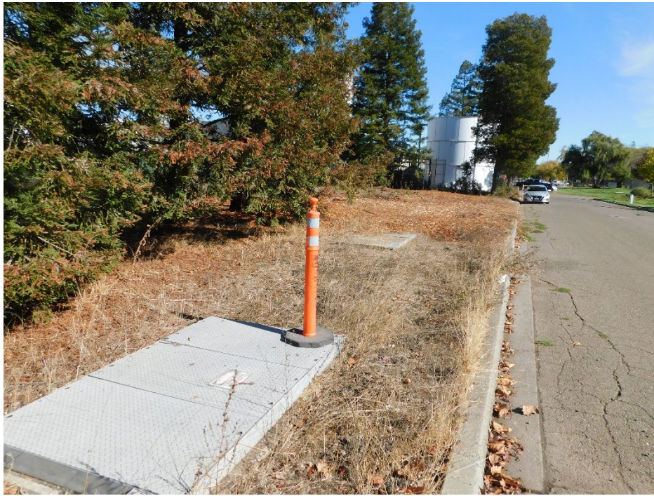
3. Photo of underground utility vault.
