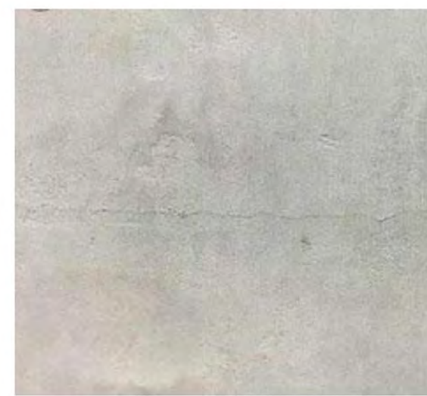
SANTA BARBARA FINISH AT EXTERIOR CEMENT PLASTER STUCCO
