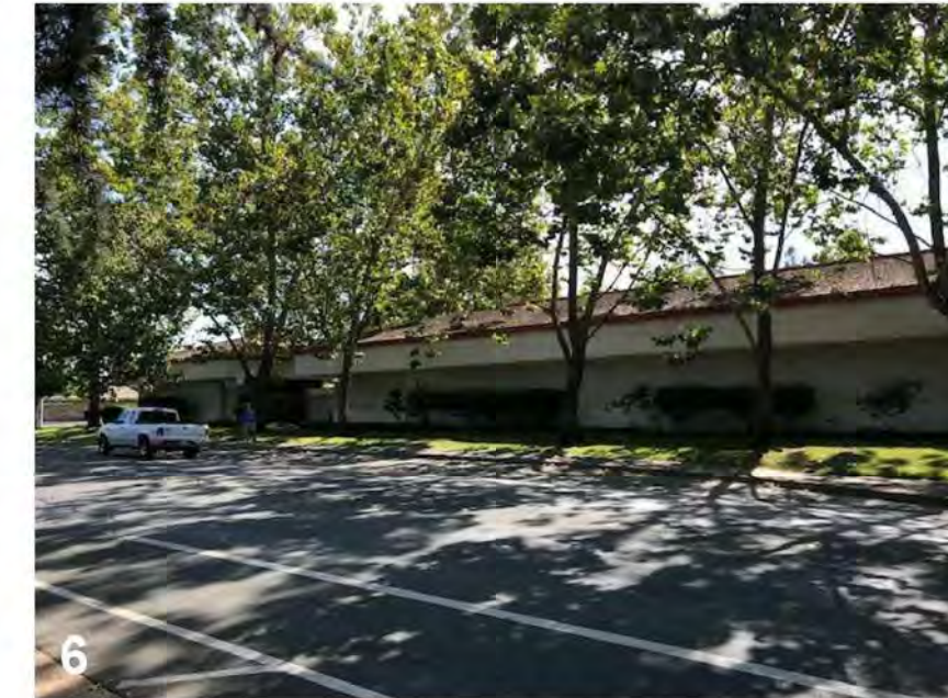
West Steele Lane Elevation of adjacent Retail
