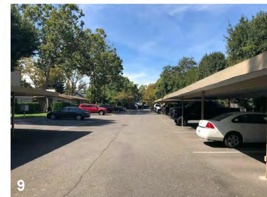
Carports at adjacent parcel at south boundary of project
