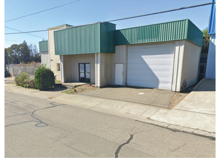
VIEW FROM NORTH EAST
