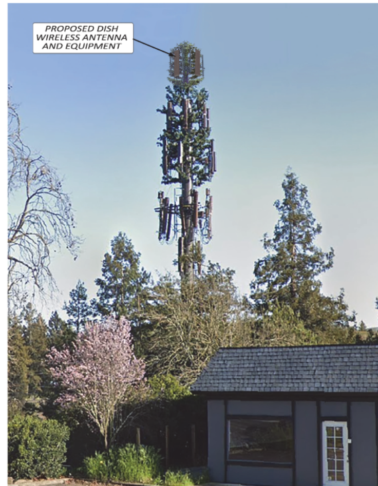
View 01-After [Looking South-East]
