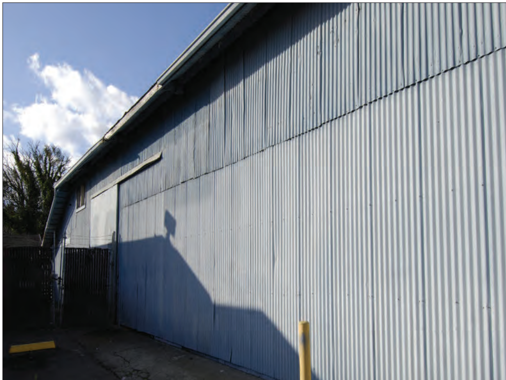
Photo 22. South façade with another sliding barn door.
