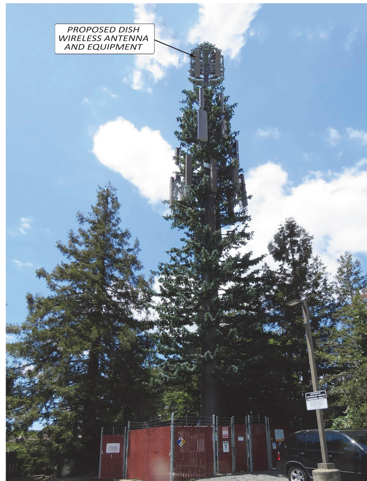
View 02-After [Looking West]
