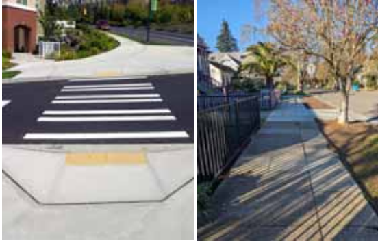
SIDEWALKS AND CURB RAMPS
