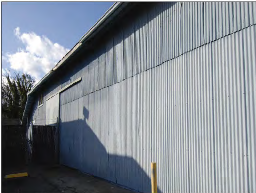
Photo 22. South façade with another sliding barn door.
