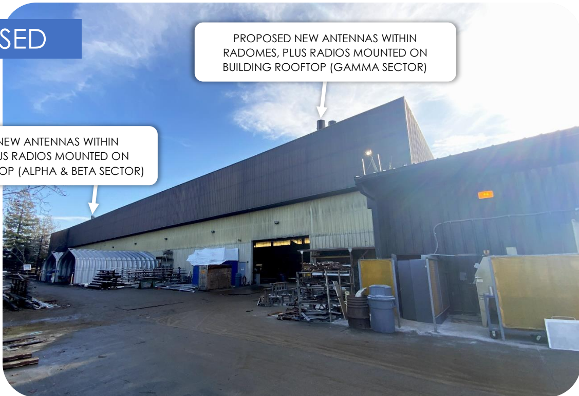
View 3: Looking southeast across parking lot | Photosim produced 03/08/2023
