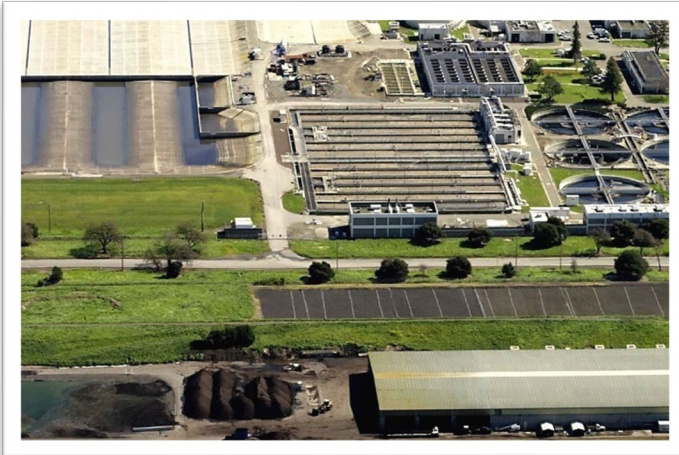
Figure 4 - Laguna Treatment Plant
