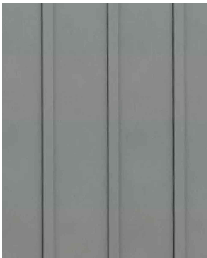
A BOARD AND BATTEN SIDING 1. JAMES HARDIE 2. SW9132 ACACIA HAZE (EGGSHELL)
