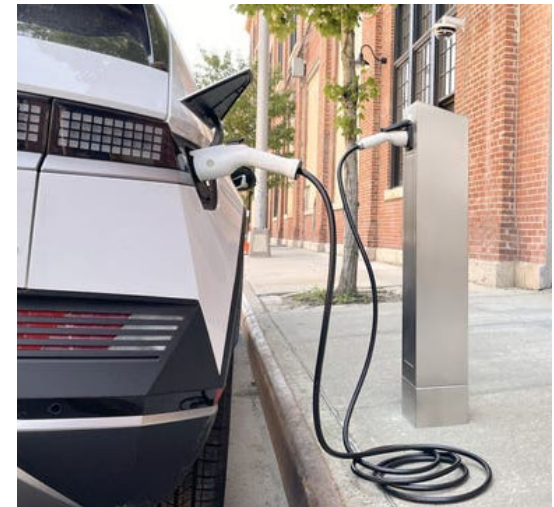
It's Electric EV Charging Station
