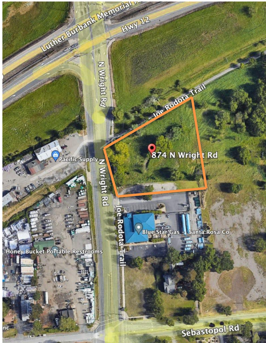
Figure 2: Project Site – Existing Conditions
