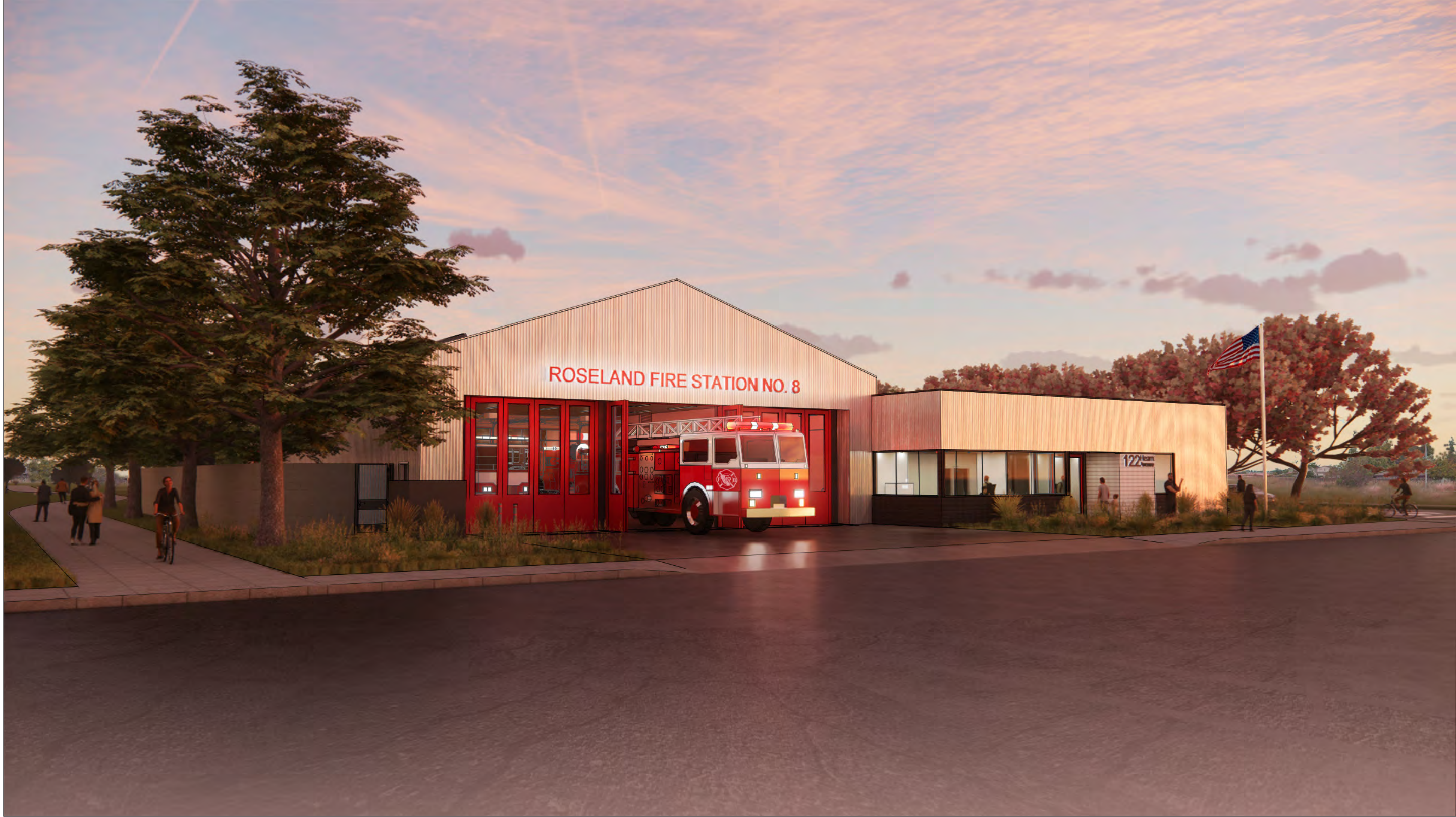
FIRE STATION FROM DUTTON LOOKING SOUTH WEST
