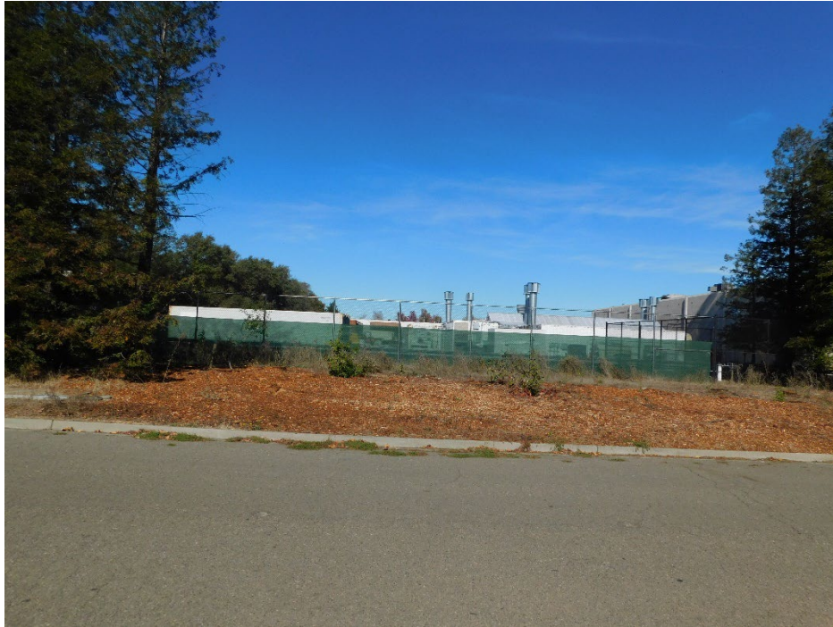
1. Photo facing north towards the parent property.
