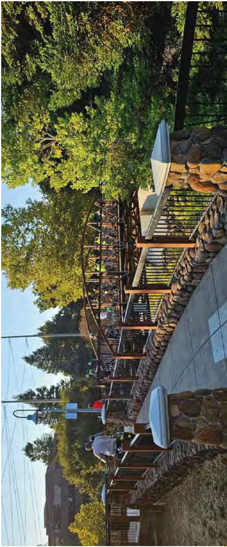
Tour de Creek bridge
