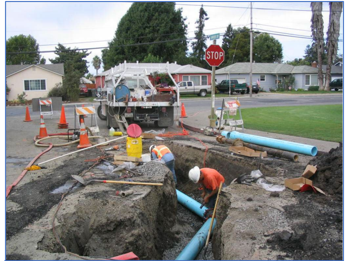
Installation of Water Distribution Main
