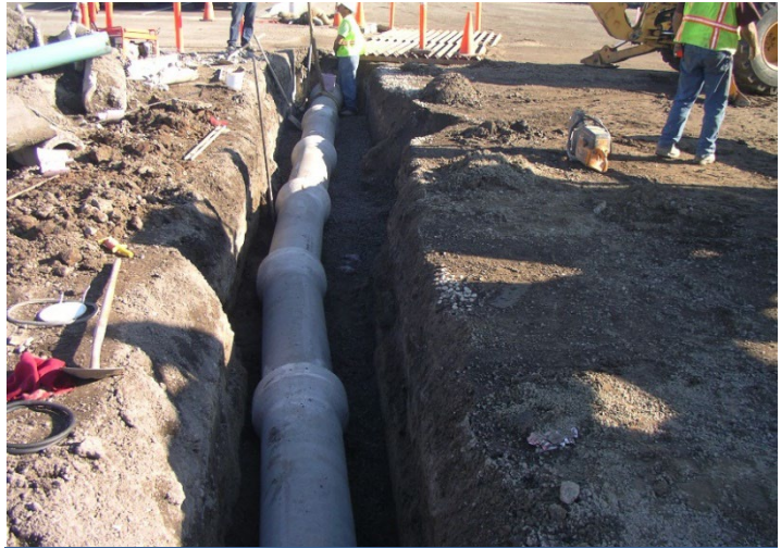
Sewer Pipe Replacement Project
