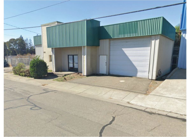
VIEW FROM NORTH EAST
