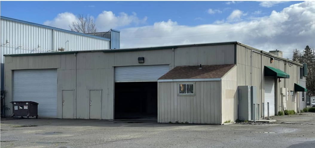
VIEW FROM SOUTH WEST
