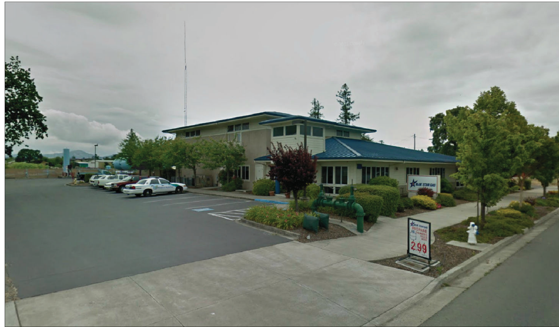
VIEW #2 SOUTHEAST VIEW at SOUTH SIDE OF SITE
