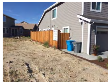
Figure 4 Wooden Fence Attached to Structure
